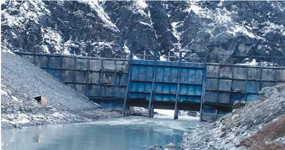
Figure 6. Tsho- Rolpa Glacial lake in Rolwaling Valley (above), sluice gate on the outlet of Tsho-Rolpa Glacial lake constructed for the purpose of lake lowering in 2000
